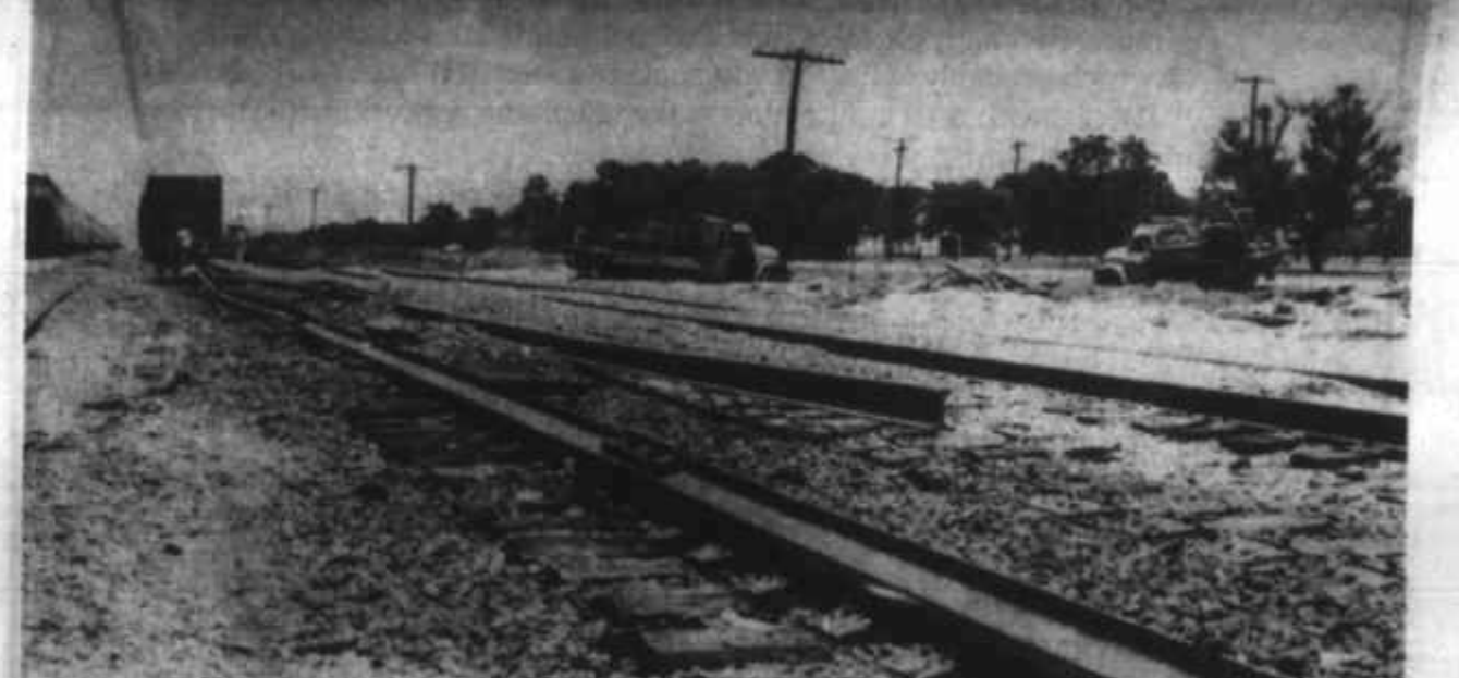
The report was available yet on the accident that tore up these rail lines over the weekend. By Sunday afternoon, workmen were repairing the tracks next to the main line along FM 102, just west of the city limits.
